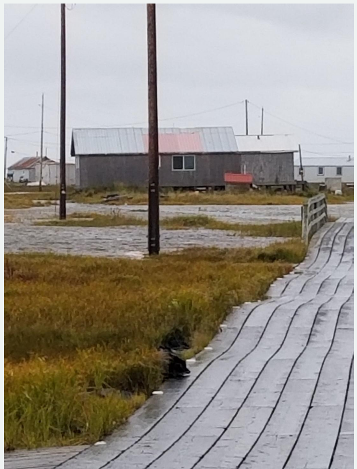
Boardwalks compromised by permafrost thaw and flooding
