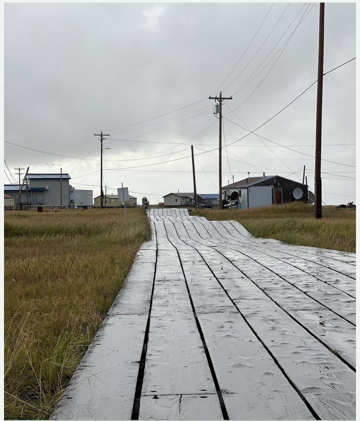
Uneven subsidence of the boardwalk is visible.
